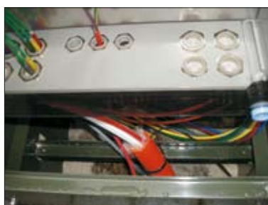
Integrated fixing bar for ducts/ tubes in root.
